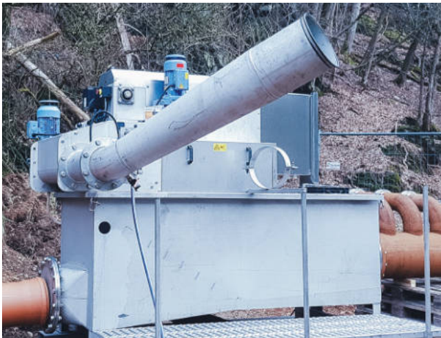
Rental screen – Flat-Fine Screen inside a container during conversion work
